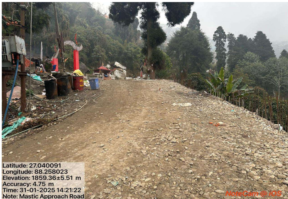
BITUMINOUS MACADAM WITH MASTIC ASPHALT APPROACH ROAD
